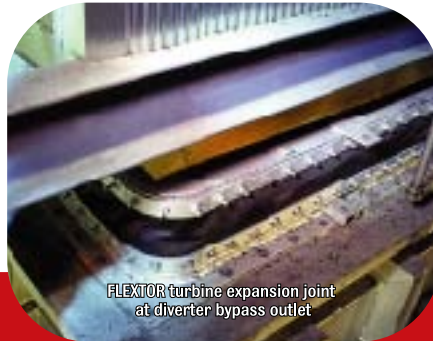
FLEXTOR expansion joint on a 600 MW SCR unit
